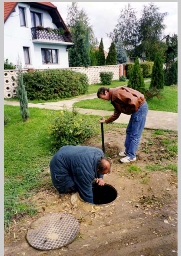
Valve Chamber Inspection
