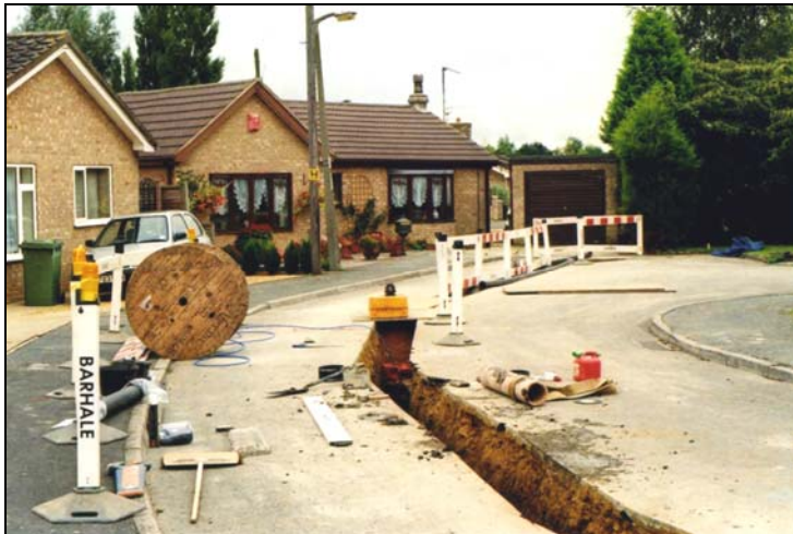
Preparation is underway for the vacuum sewers to be laid
