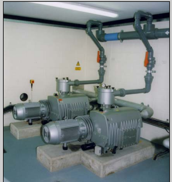
630m 3 /hr vacuum pumps installed
