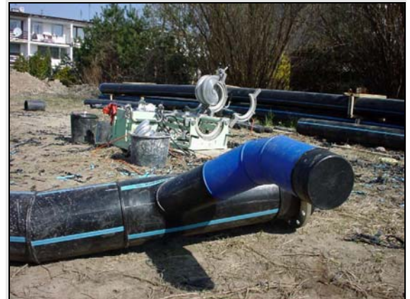
Sewer junctions being fabricated
